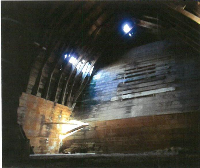
Left: The loft of the barn, where hay was stored. Holes in the roof are evident here. Above, the cupola, part of the venting system. Below, a full view of the front, complete with silo.
